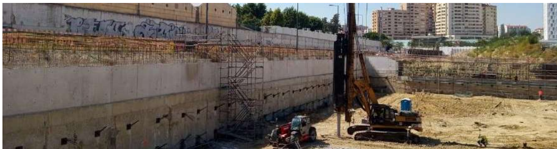
Figure 4 Pile Driving Analyser preliminary tests being executed at Lot 2.
