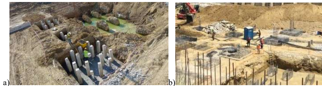
Figure 12 a) and b) show the execution of the foundations at Lot 2'.
