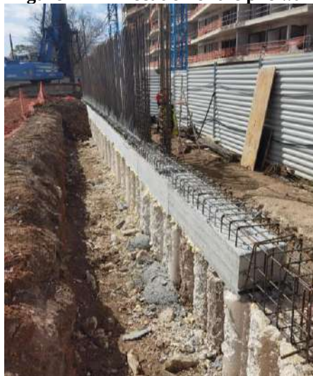
Figure 15 - Secant pile wall
