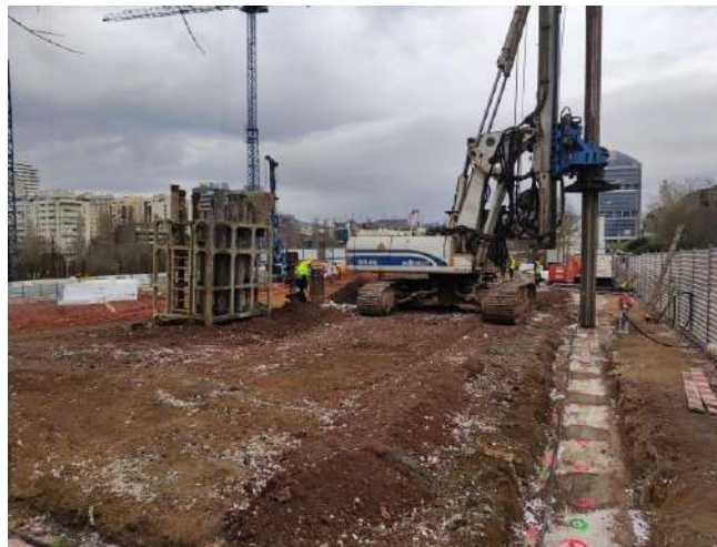
Figure 14 – Execution of the pile wall
