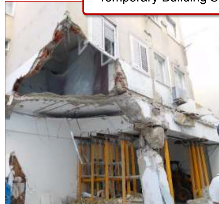
Temporary Building Shoring
