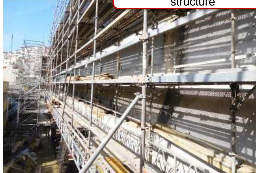
Scaffold suspended structure
