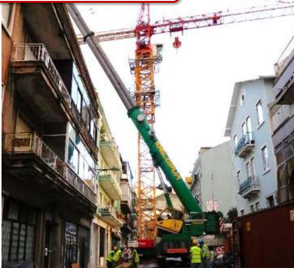
Tower crane installation on the adjacent street
