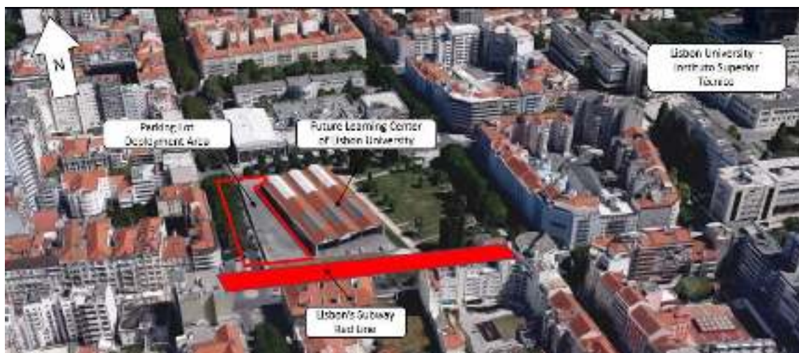
Figure 1. Excavation site and surroundings. Source: adapted from Google Maps
