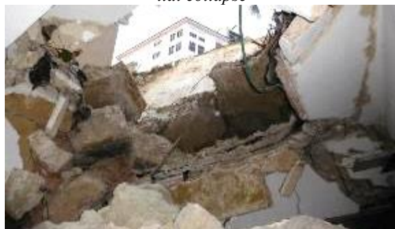
Figure 3. View from building n.º106 basement after earth retaining walls partial collapse
