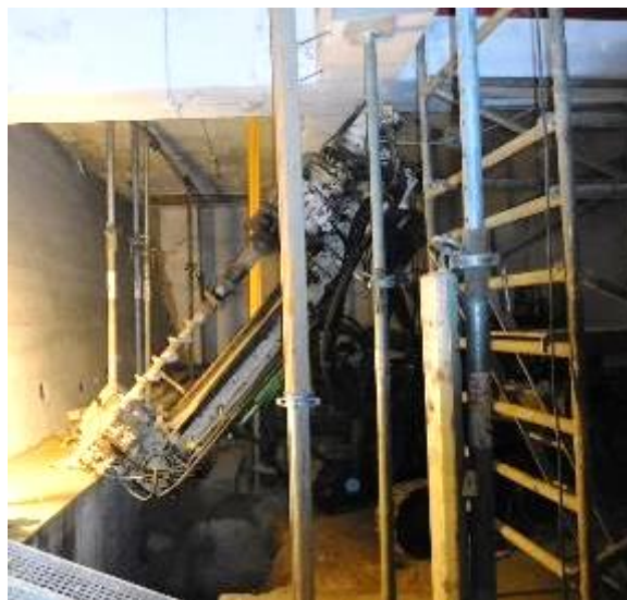
Figure 9. Micropile equipment inside building basement
