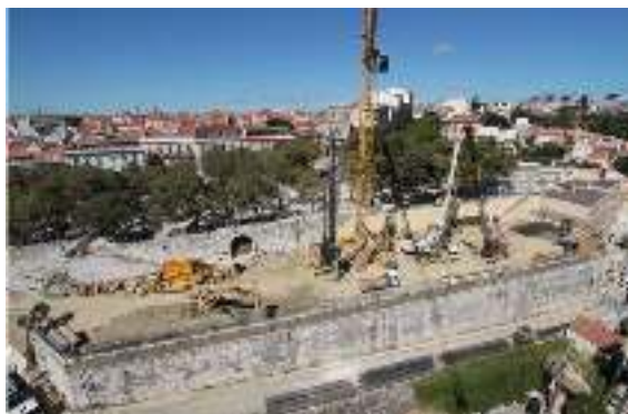
Figure 8. View of the piles works.
