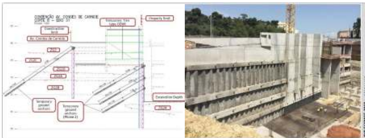
Figure 3. Section Cut and Construction Works
