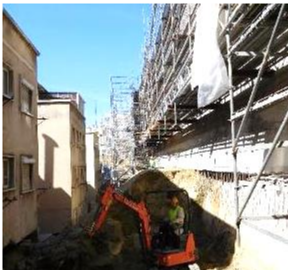
Figure 10. Climbing scaffolding and works bellow
