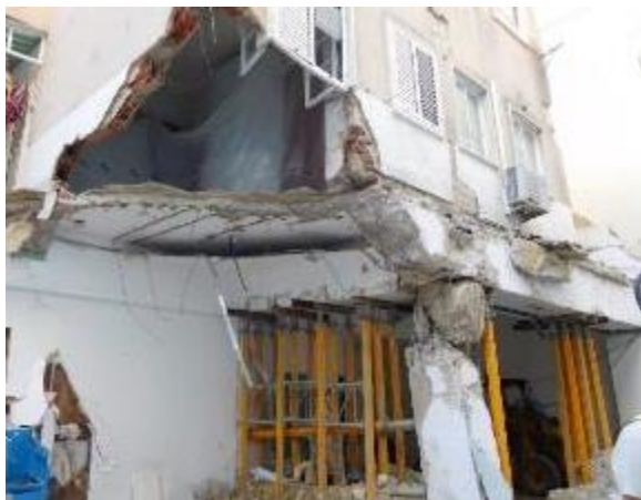
Figure 4. View of building n.º108 basement shoring
