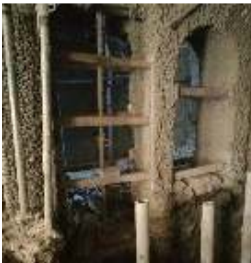
Figure 2 - Shoring of the arches and installation of steel props (September 2018)
