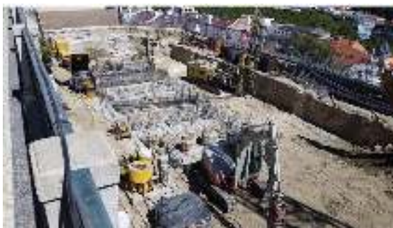
Figure 10. View of the nail's execution.
