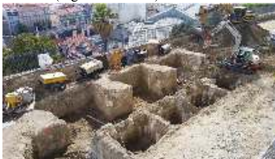
Figure 9. View of the excavation works.
