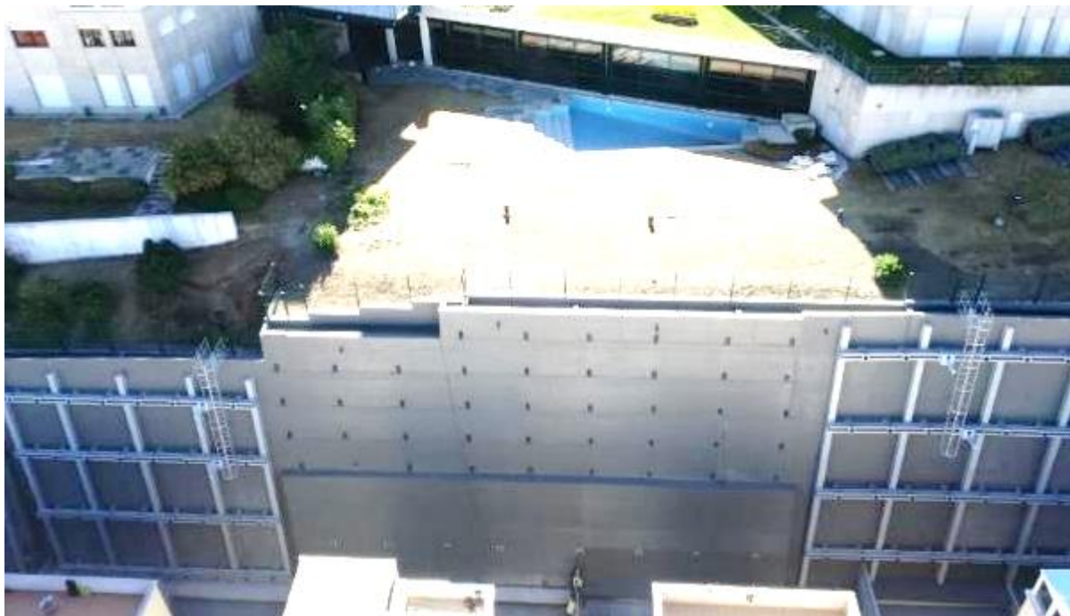
Figure 13. View after final works
