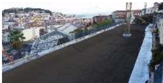
Figure 12. View of the final works
