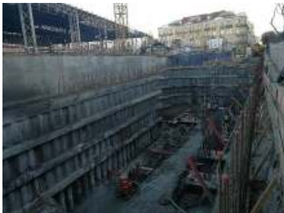
Figure 8. View of the final excavation works.
