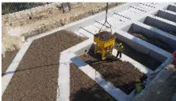
Figure 11. View of the lightweight aggregates
