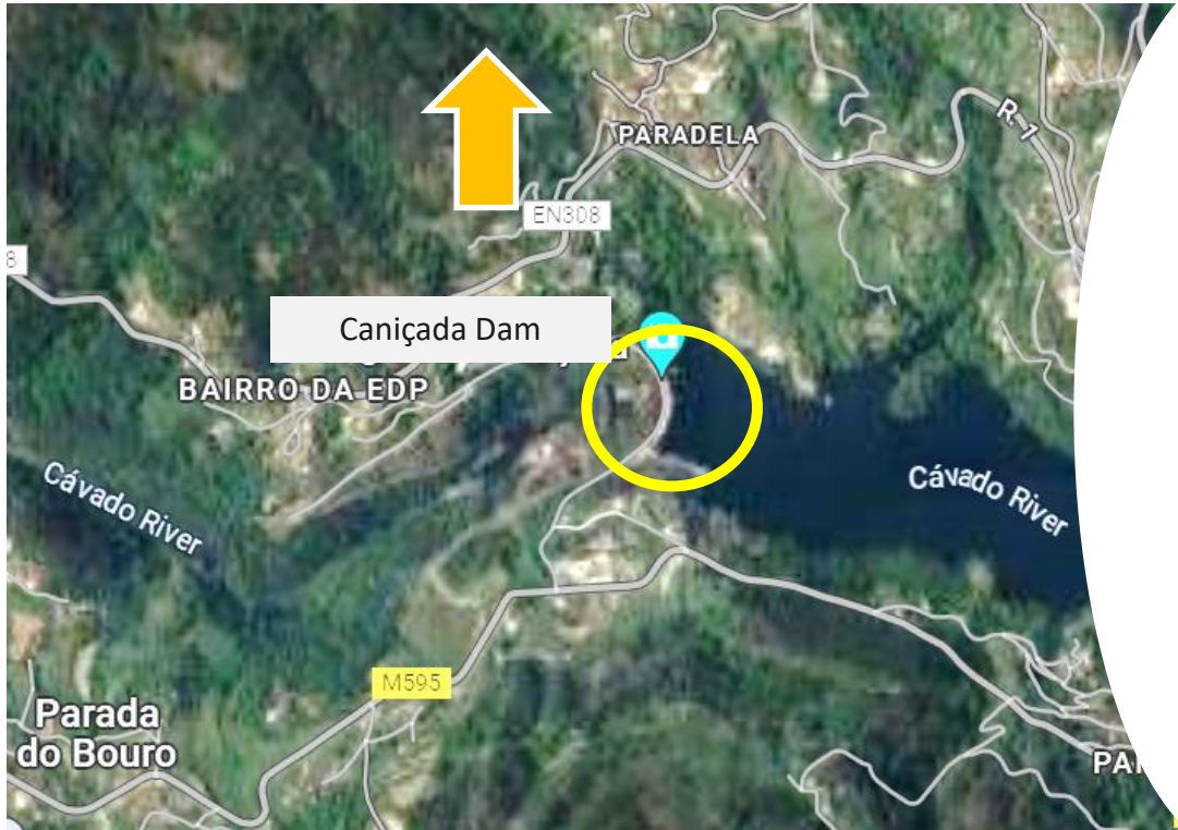
Caniçada Dam location
