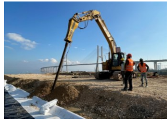
Ductile iron piles driven
