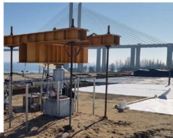
Pile compression full scale load test
