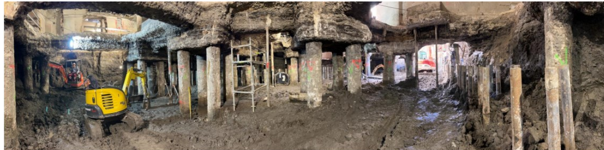
Excavation work in the area of the existing foundation piles
