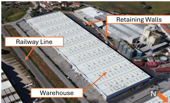
Overall view before intervention
