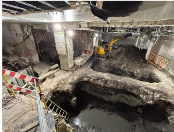
Execution of jet-grouting columns
