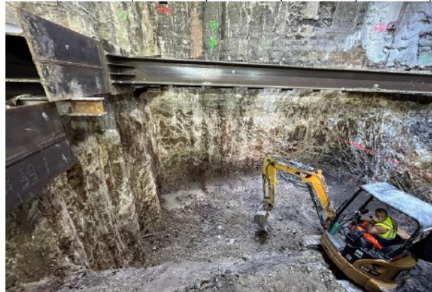
Installation of the fourth level of steel struts
