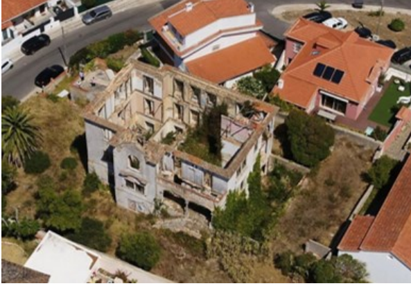
Overall view before intervention
