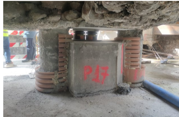
Sheathing of the piles
