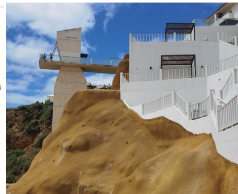
Rock cliff after intervention
