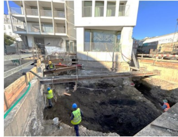
Installation of the first level of steel struts
