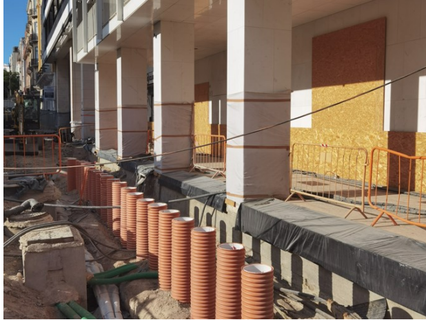
Execution of jet-grouting columns
