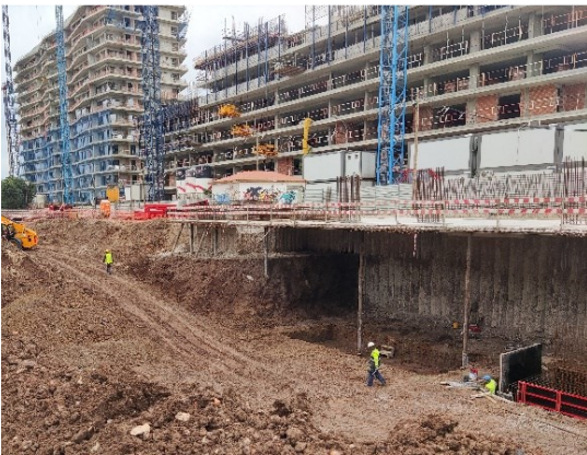
West side excavation works (under slab band)
