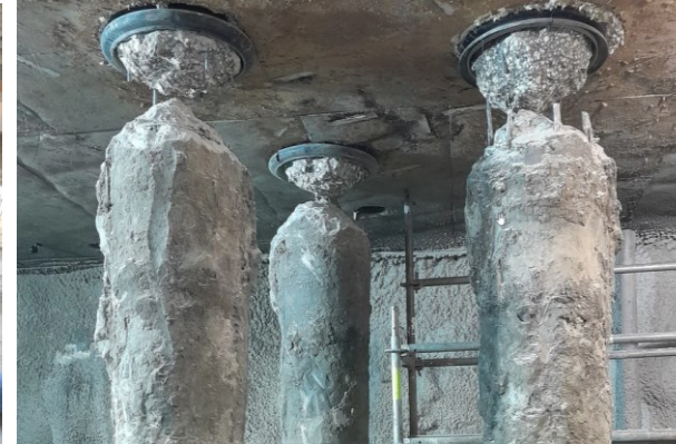
Demolition of the piles
