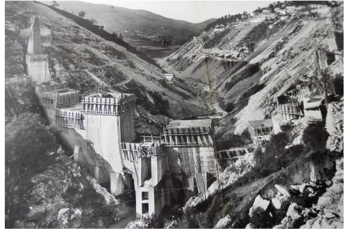
Caniçada Dam construction (1955)
