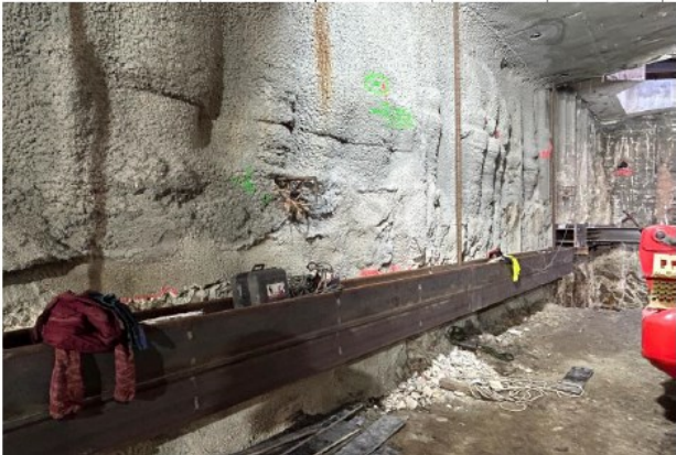
Second and third strut level in the pile wall and in the diaphragm wall section
