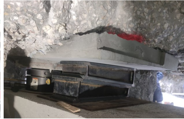
Fitting temporary chocks
