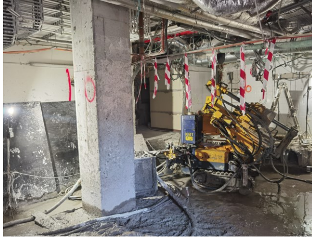
Execution of jet-grouting columns
