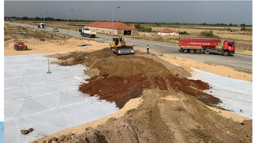
Preload embankment construction over drainage geocomposite
