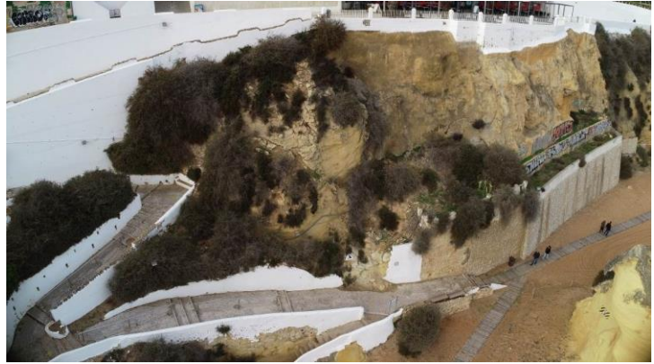
Overall view before intervention
