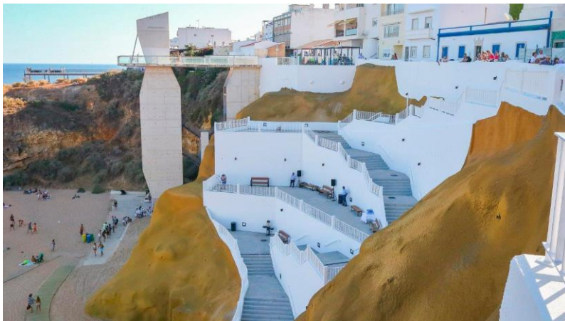
Overall view after intervention
