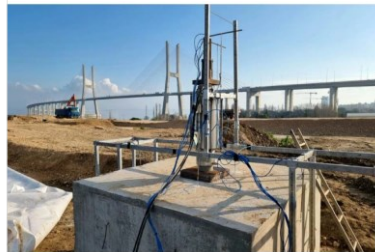
Pile tension full scale load test
