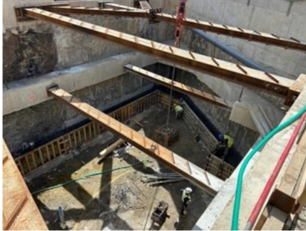
Second and third strut level in the pile wall and in the diaphragm wall section
