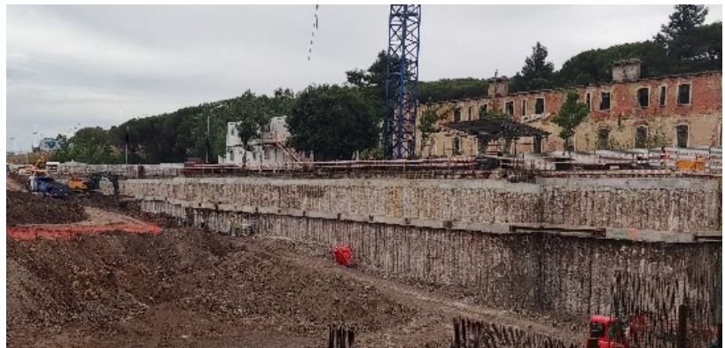
East side excavation works
