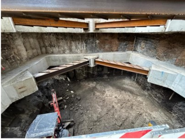
Second and third strut level in the pile wall and in the diaphragm wall section
