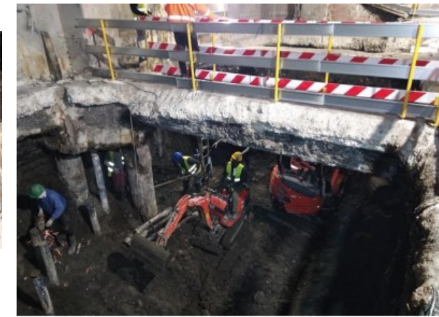
Installation of the first level of steel struts
