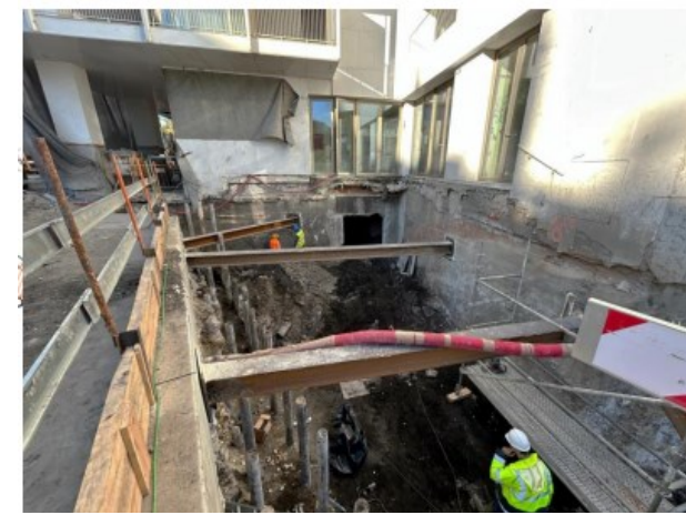
Installation of the first level of steel struts
