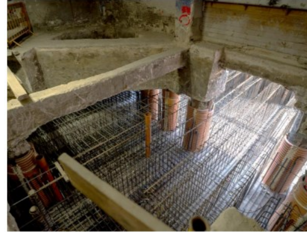
Steel reinforcement of the slab
