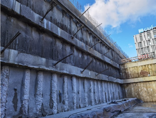
Figure 5 - Bored pile wall shored temporarily by ground-anchors.
