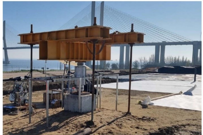
Figure 13 - Reaction structure for the compression load test.
