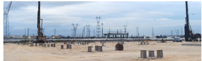
Figure 2. Driven piles.
