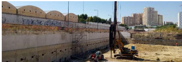
Figure 6. Pile Driving Analyser preliminary tests being executed at lot 2.
