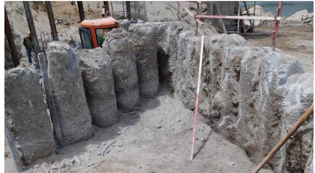
Figure 12. View of jet grouting excavated around columns.
