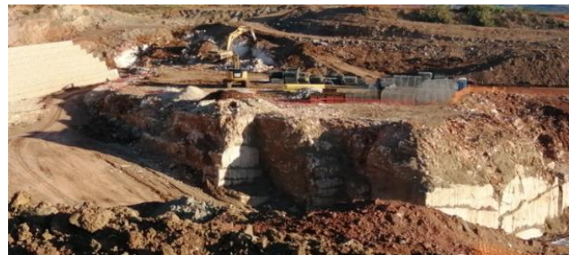
Figure 3 - View of abrupt transitions between landfill zones and vertical faces of the limestone quarry.
