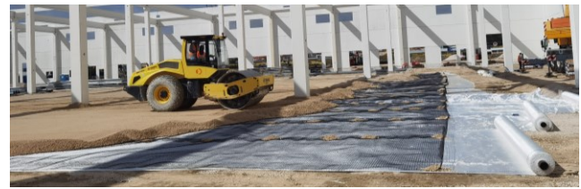
Figure 5. Load transfer platform.
