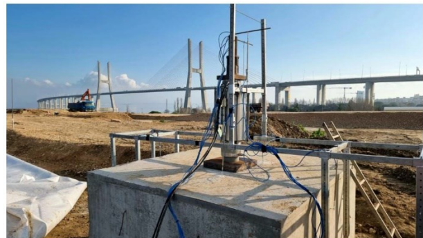
Figure 10 - Tension load test.
