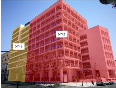
Figure 1. Reinforced concrete buildings above de tunnel.
