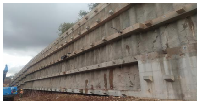
Figure 6 - Excavation works near the bored pile wall.
