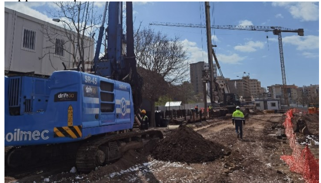
Figure 10 - East Side with 2 pile machines.
