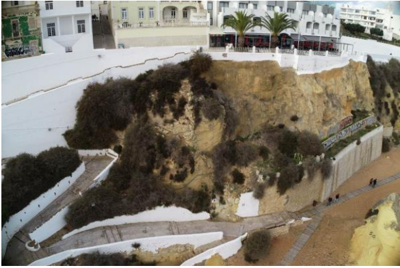
Figure 1. Cliff before intervention.
