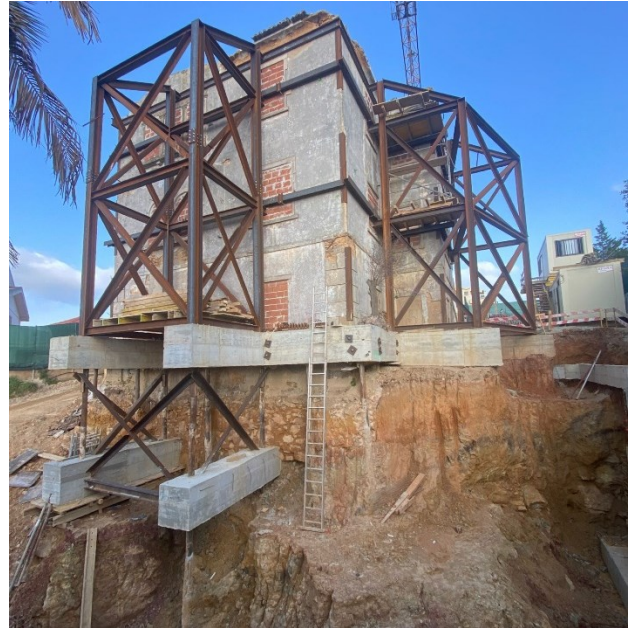
Figure 5 - Facades retention and underpinning solution.
