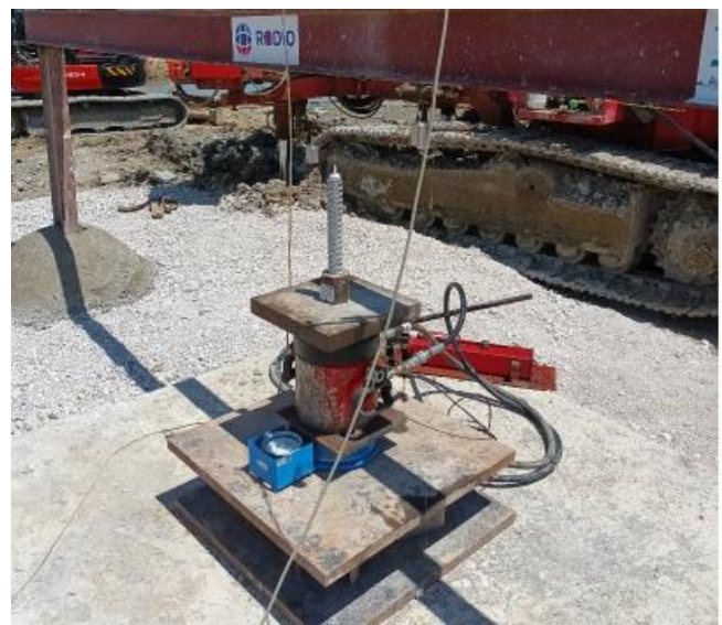
Figure 7. Full scale tension test: reaction structure view.
