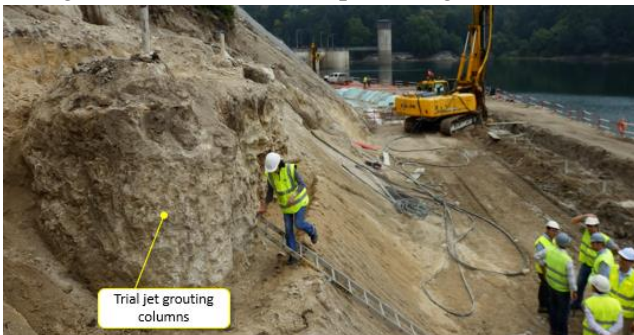
Figure 11. Trial column's view.
