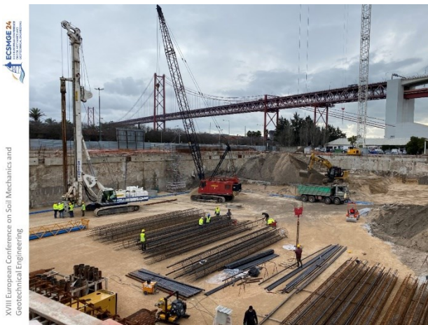
Figure 7 – Excavation works at 6.0m depth.
