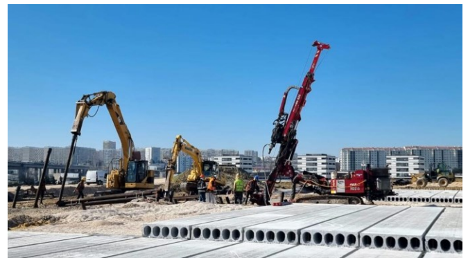
Figure 6 - Precast hollow-core slabs.
