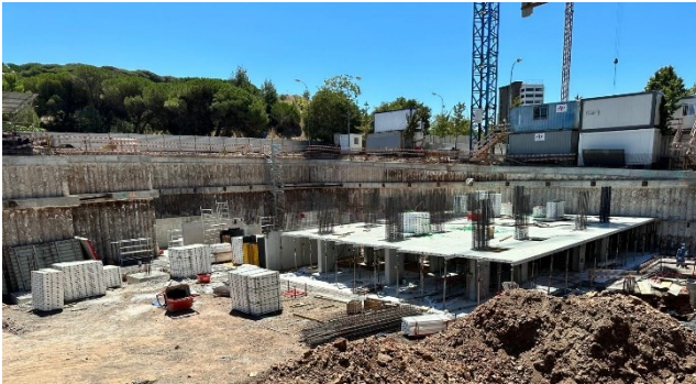
Figure 13 - South Side solution with provisory anchors. (definitive structure already in place).
