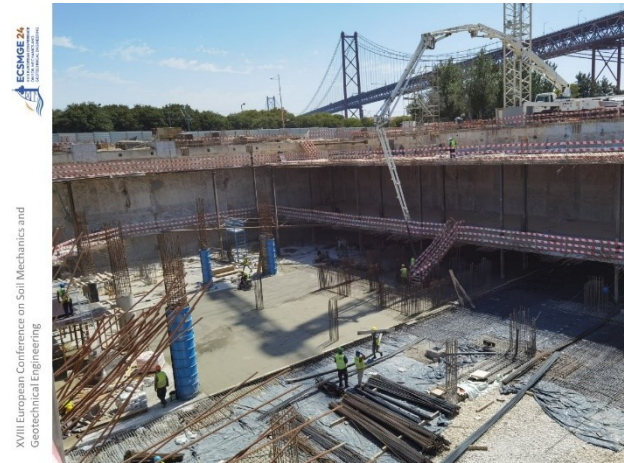
Figure 13 – Bottom drainage gravel layer.
