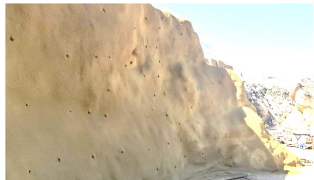
Figure 5. Cliff's surface after intervention.
