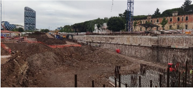
Figure 12 - East Side solution with provisory anchors.
