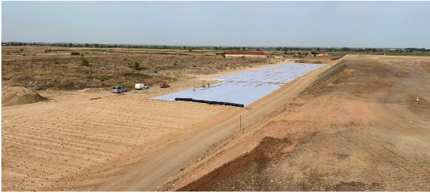
Figure 4. Aerial photograph of the drainage geocomposite installation.
