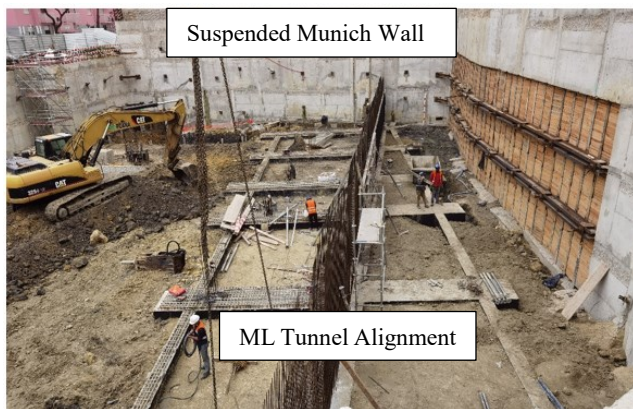
Figure 7 - Plot 1 – Suspended Munich Walls.
