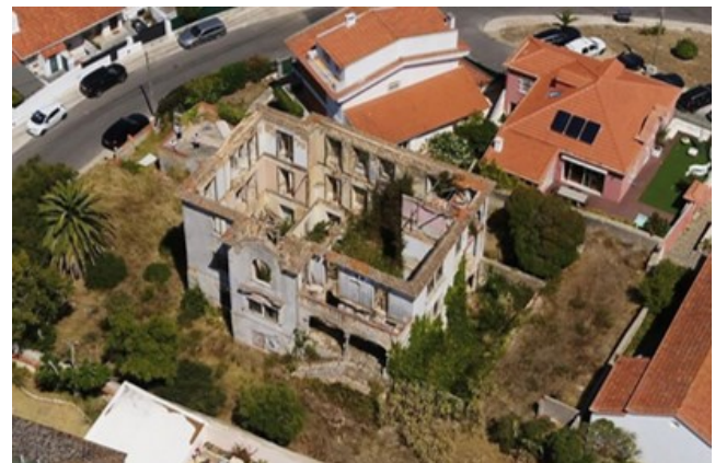
Figure 1 – Aerial view of the intervention site, in its current state.
