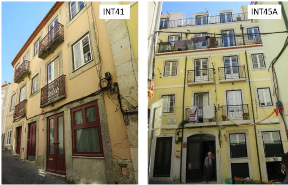
Figure 1. Centenary buildings located above de tunnel.
