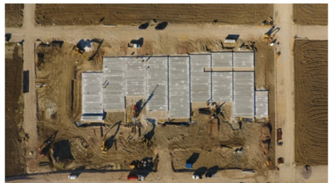
Figure 7 - Top view of the spread foundation of the stage already assembled.
