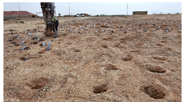
Figure 3. Installation of the prefabricated vertical drains.
