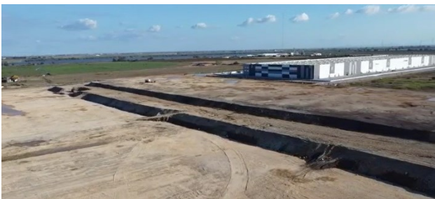
Figure 5. Aerial photograph of the preload embankments.
