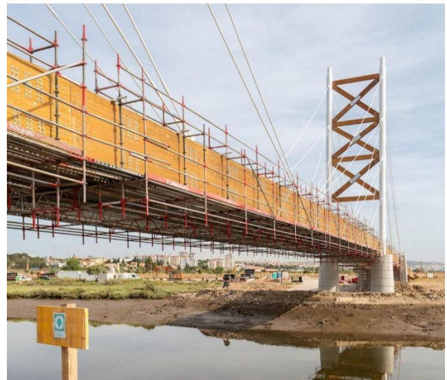
Figure 10. Bridge view just before the YWD, August 2023 with the deck being reinforced for the pope's car crossing.
