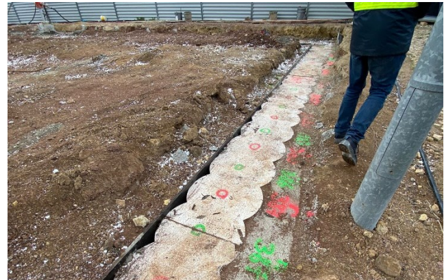
Figure 4 - Overlap pile wall preparation in situ with marks.
